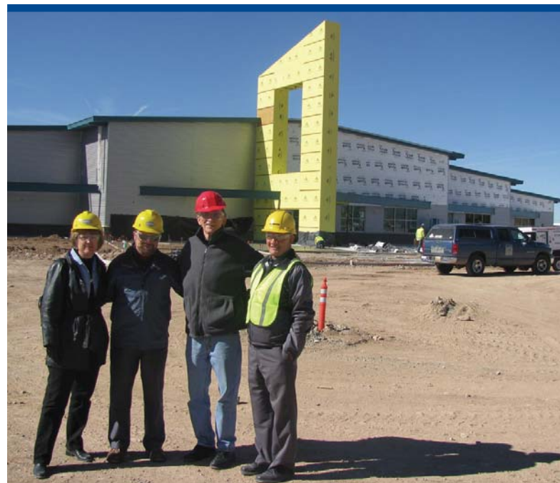
NUCLEAR SCIENCE REPOSITORY: New construction for the relocated National Museum of Nuclear Science and History (formerly the National Atomic Museum), chartered by Congress and located in Albuquerque, N.M., is scheduled for completion in March 2009. The 30,000 square foot facility will incorporate 13 permanent indoor exhibit areas, two classrooms, a theater, library and conference room, a gallery for temporary exhibits, and the museum's store. The site provides nine acres of outdoor space for exhibits of military aircraft, missiles, vehicles, and the sail of the USS James K. Polk nuclear submarine. Touring the site are (left to right) NNSA Service Center Director Karen Boardman, Service Center Deputy Chief Counsel Rick Vergas; former Albuquerque Operations Office (ALO) Deputy Manager Jim Culpepper; and National Atomic Museum President, construction project manager, and former ALO employee Chuck Loeber.
